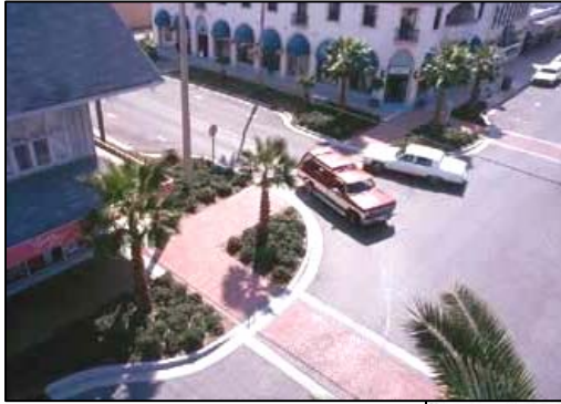
Photo and diagram illustrate features of pedestrian bulb-outs
